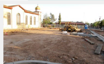
The parking lot addition is taking shape!
